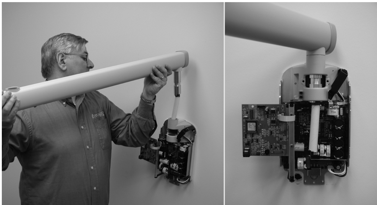
Figure 18 Installation du bras horizontal
